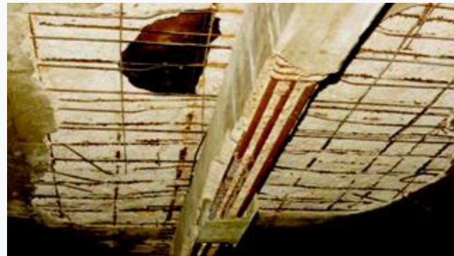
Rebar corrosion
